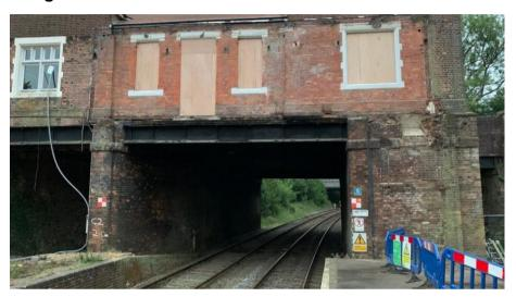
Vital work to remove and reconstruct a footbridge at Eridge station in East Sussex took place over the weekend. The work was needed due to the age and condition of the old structure, in order to protect the safety of those using the bridge and the trains operating below. The existing staircases and bridge are being replaced with a new modern-designed footbridge.
